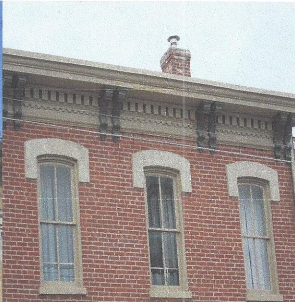
BRACKETS & DENTILWORK+"EYEBROW" LINTELS
